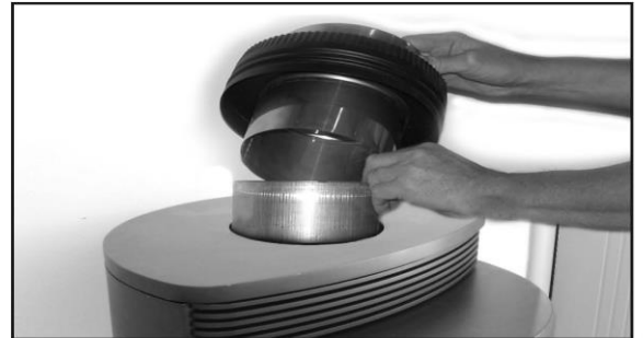
Start by fitting the adapter pipe,using stove sealant (see photo).The next stage is to fit the connection piece and the flue modules,in accordance with the chimney manufacturer's instructions
