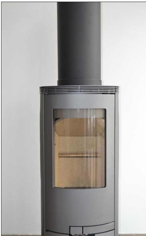
Ellipse 2 in black ,top connected and ready to be inspected by the chimney sweep.
