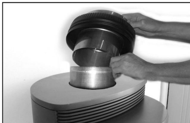
Start by fitting the adapter pipe, using stove sealant (see photo). The next stage is to fit the connection piece and the flue modules, in accordance with the chimney manufacturer's instructions
